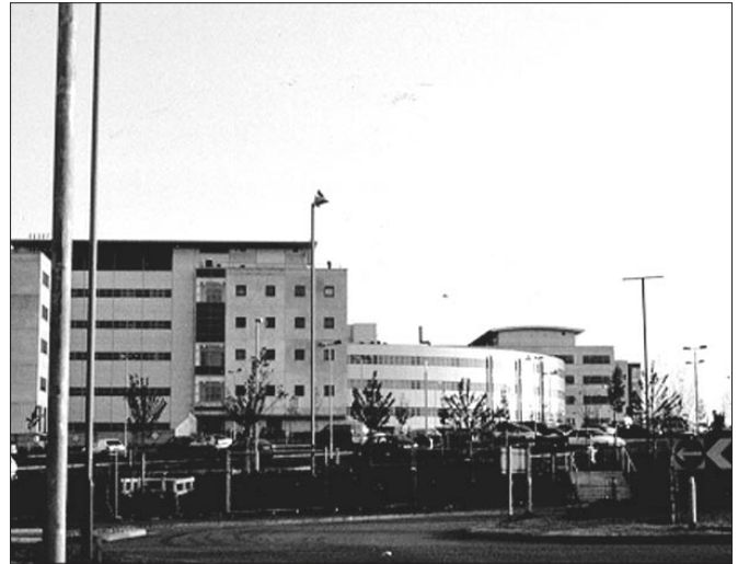
Big corridors ... shame about the lack of office space: Swindon's Great Western Hospital
