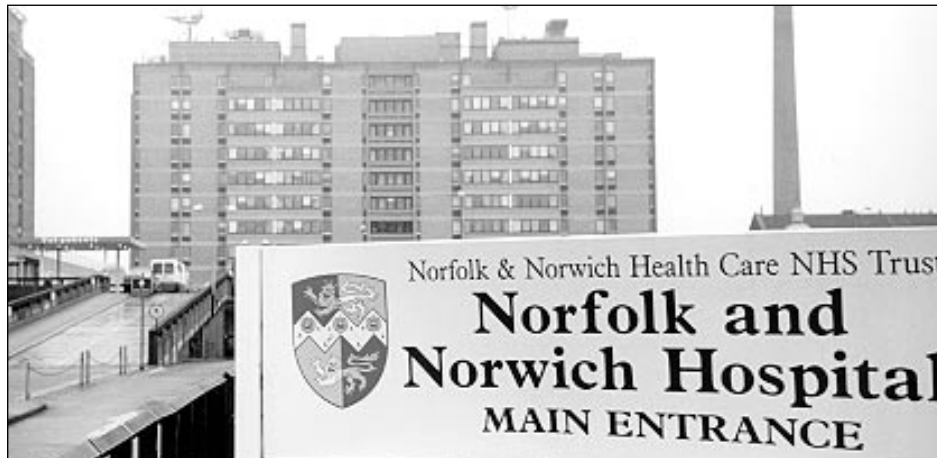
The PFI-funded £228m replacement for the Norfolk & Norwich Hospital is on a greenfield site on the edge of the city, and will cost £33.5m a year for 30 years.
