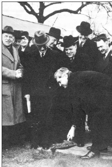
1948: Nye Bevan lays a foundation stone for a new health centre: but capital investment was minimal in the early years of the NHS
